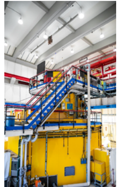
Overview of the reactor block with biological shield
