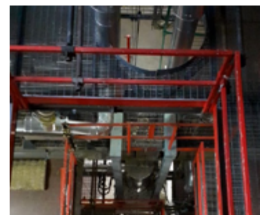
SIRIO facility: tests on a passive DHR system for the ALFRED LFR
