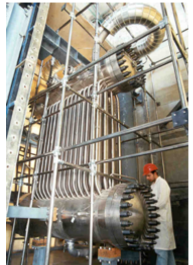
SBWR Isolation Condenser testing on the PANTHERS facility (power: 20 MW)
