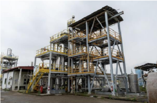
Internally circulating fluidized bed - Air/O 2 /steam 1MW th
