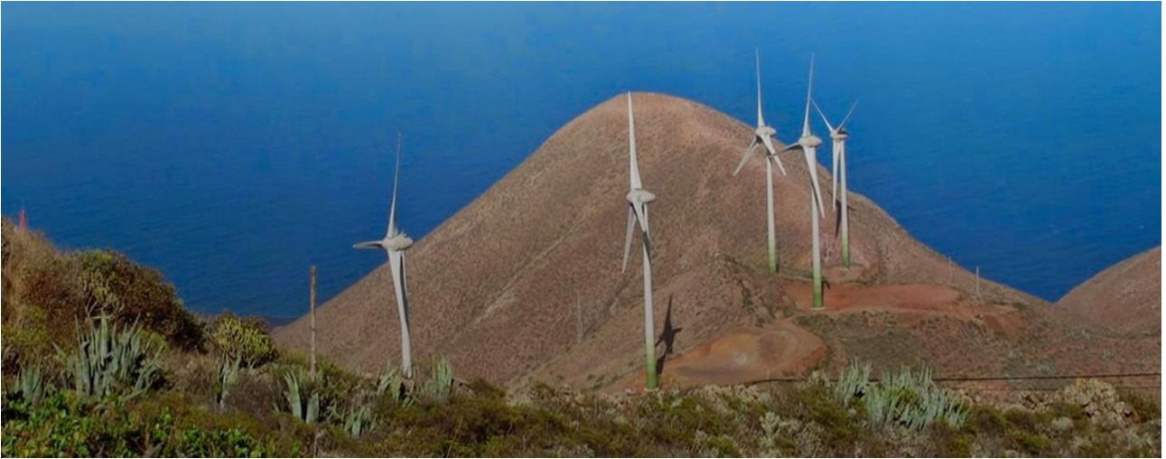
Wind farm in El Hierro, island of the Canary Archipelago
