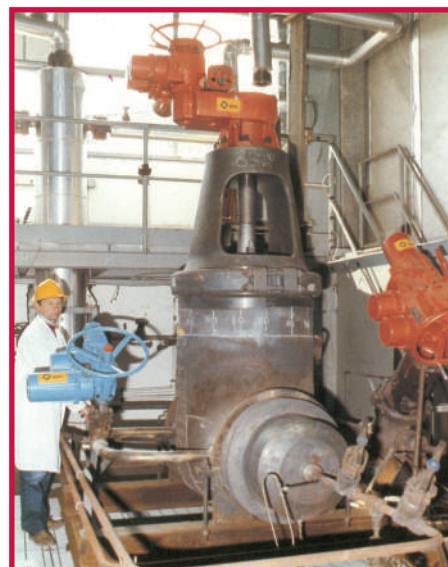
Pressurization tests on an isolation valve
