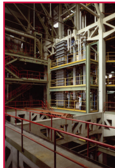
SPES-2 experimental facility: North side view, passive safety system (total height: 30 m)
