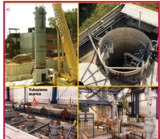
VAPORE plant building site:
