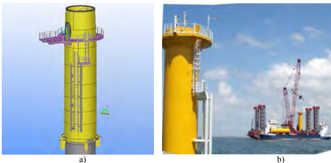
Figure 5: Transition piece in a functional representation (a) and during installation (b).
