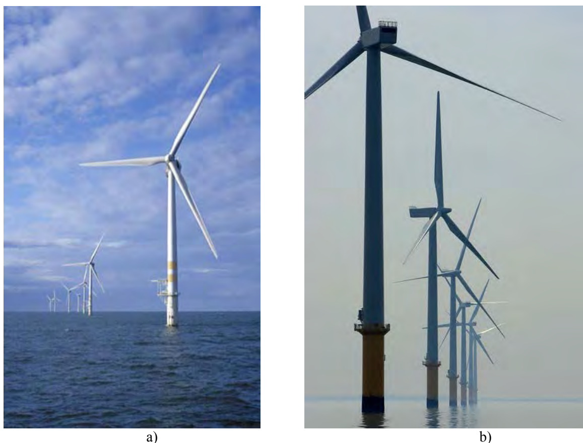
Figure 3: Turbine monopile substructure in english windfarms: Arklow Bank (a) and Burbo Bank (b).
