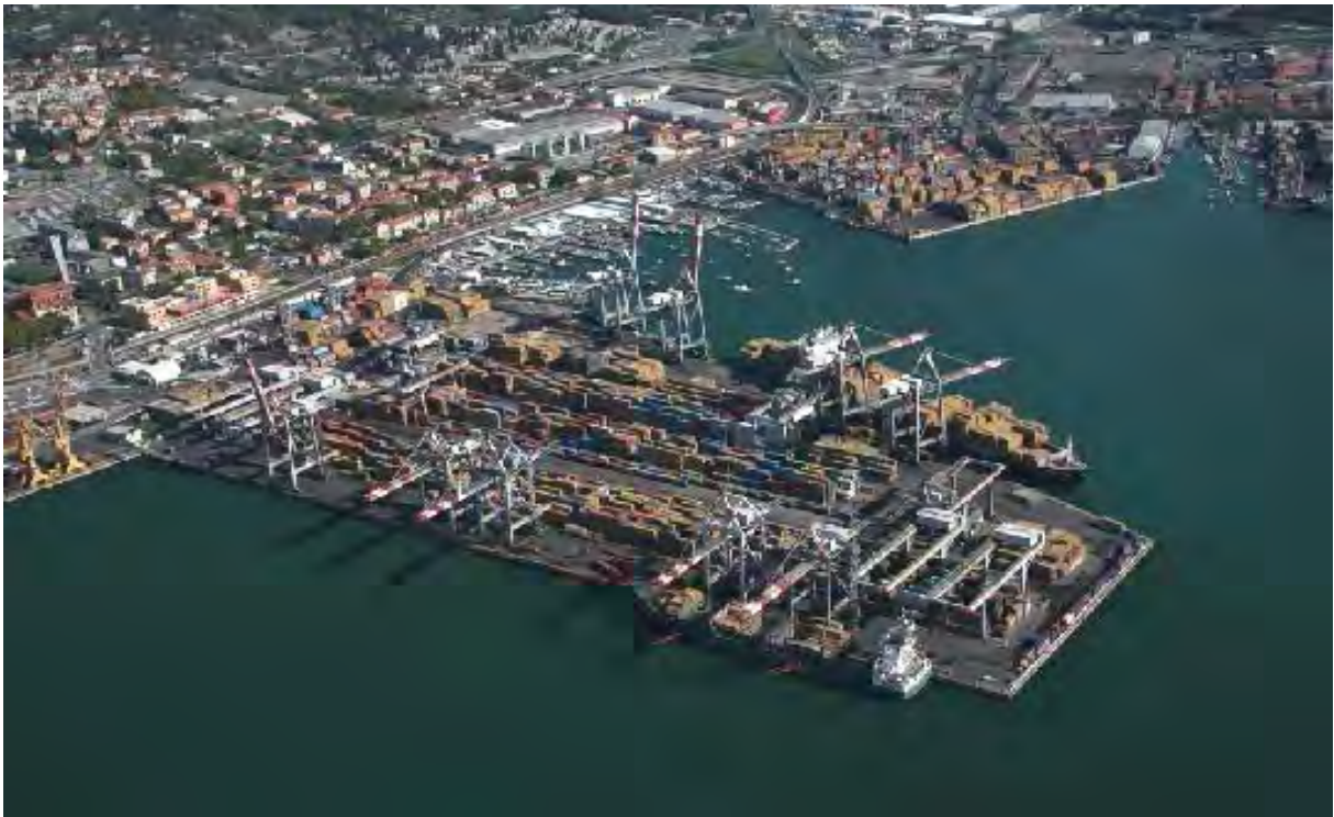
Figure 3: Quay in the Port of Gioia Tauro.
