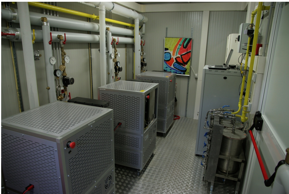
Figure 36. "Isola Cogenerativa" is the first SOFC cogeneration plant in Italy; it consists of 3 modules of 1 kW e fueled by natural gas, for a total of 3 kW of electricity and 6 kW of heat for domestic hot water.
