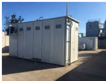
Fig. 2. Installation of the complete system at GE's site in United Kingdom.
