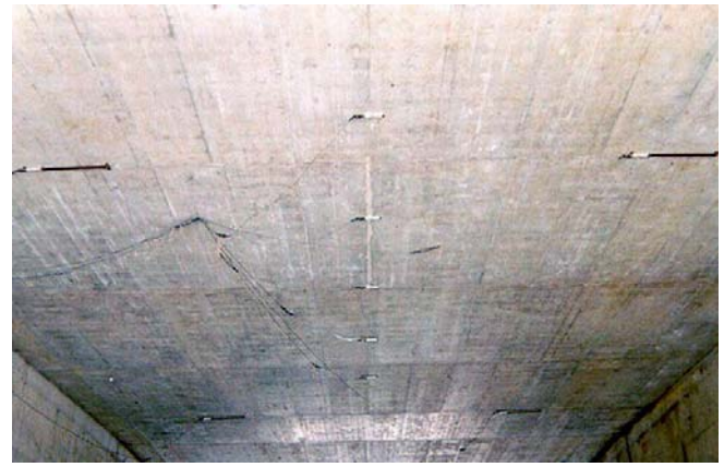
Figure 3. FAD bridge WIM installation.
