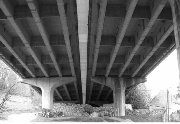
Figure 5: View of the girders of Roberval bridge
