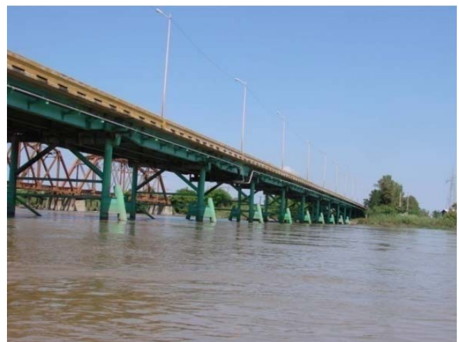
Figure 1. Panoramic view of “El Prieto” Bridge.
