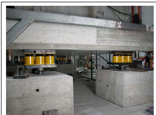
Figure 12: Series of Gerb steel springs under the concrete slab
