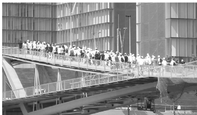
Figure 8: Field tests on the Simon de Beauvoir footbridge (after OTUA 2008)
