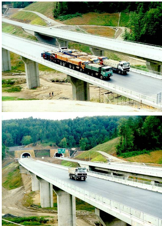
Figure 8. Diagnostic load test with pre-weighted vehicles, static (above) and dynamic with one vehicle (below).
