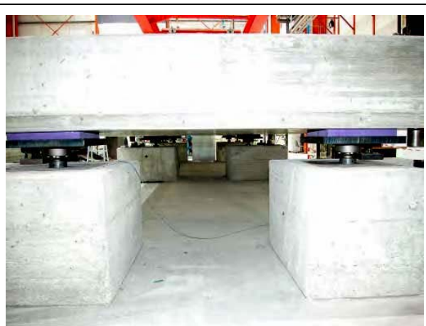
Figure 9: Getzner bearings (violet) placed under the concrete slab
