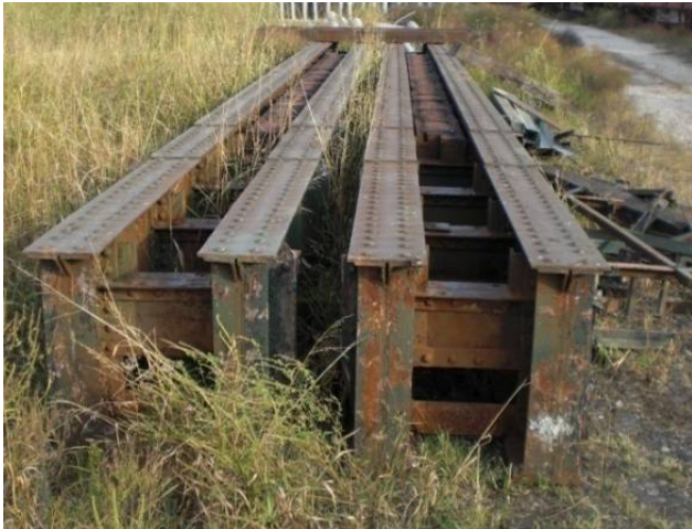
Fig. 4: Twinned beams after dismantling.
