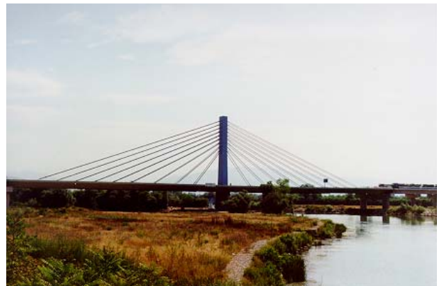
Figure 2. The Garigliano Bridge
