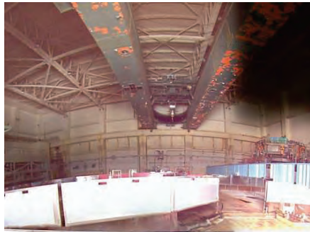
Unit-2 5th Floor ( Operating Floor)
