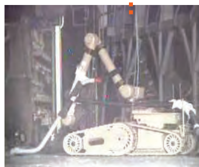
Cleaning in Reactor Building of Unit 3 (July 1)
