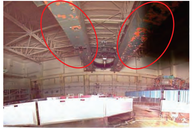
Situation of 5 th floor of reactor building with no steam release (photo as of Oct. 20)
