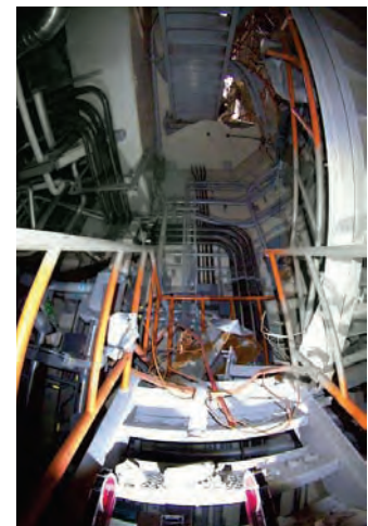
Unit-3 Stairs to 3rd Floor in R/B
