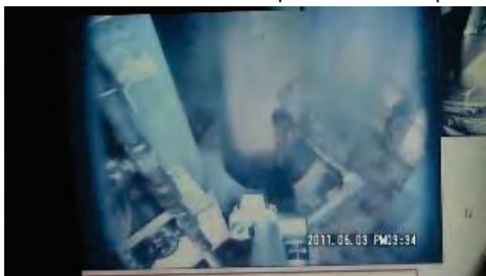
Steam release from the penetration on 1 st floor (photo as at Jun. 3)
