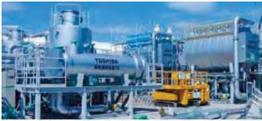
Evaporative concentration apparatus (3A, 3B, 3C)
