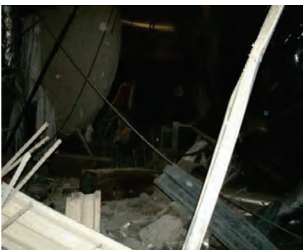
Unit-1 Isolation Condenser Room
