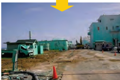
Removal of debris
