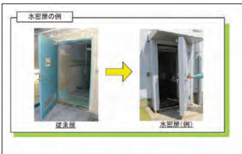
Watertight door (Source: The Shikoku Electric Power Co.,Inc.)
