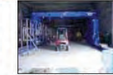
③ Installation of lifter for changing adsorption towers
