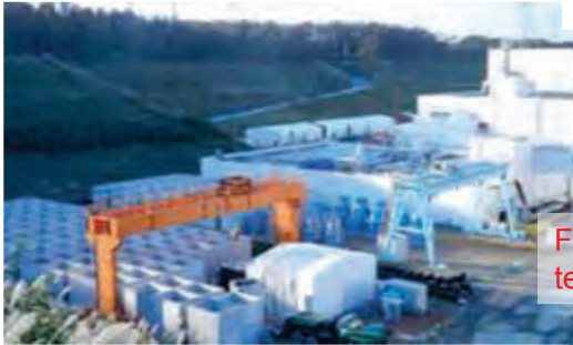
Current facility for secondary waste storage after water treatment
