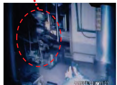
Surveying high dose area in Turbine Building of Unit 1 (August 2)
