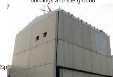
Unit 1 reactor building cover installation
