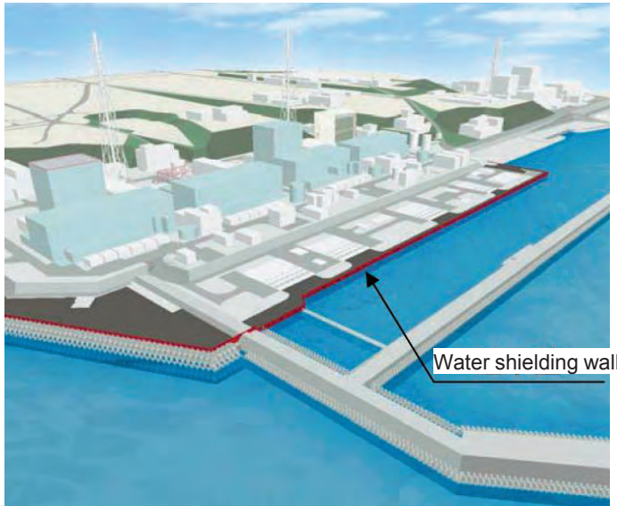
Image of water shielding wall
