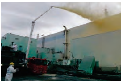
Spraying dust inhibitor agents to the buildings and site ground
