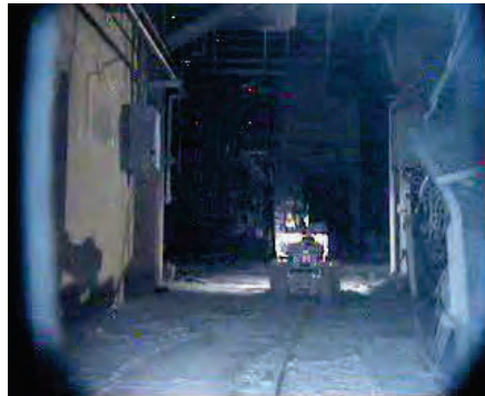
Unit-3 West Aisle in R/B 1st Floor
