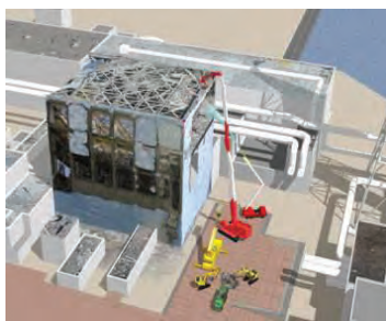
Debris removal from the upper part of reactor building
