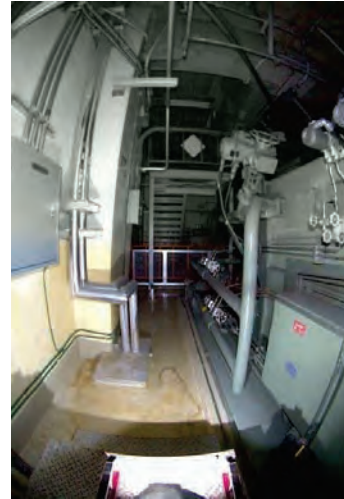
Unit-2 Aisle on 3rd Floor in R/B
