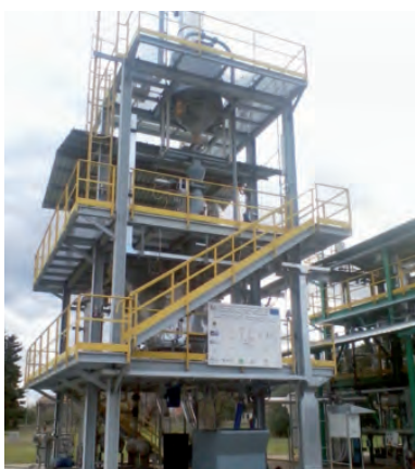
Different types of biomass gasification plants at the ENEA Trisaia Research Centre
