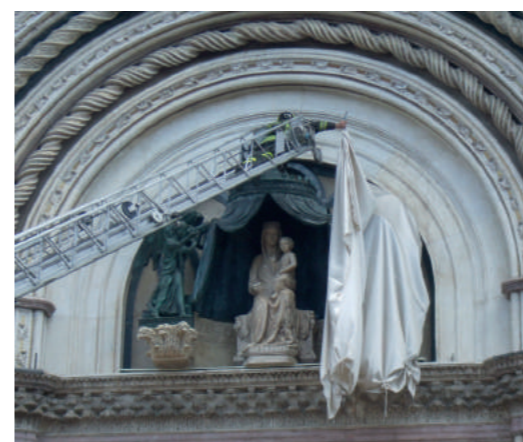
Repositioning of the Maestà on the façade of Orvieto Cathedral
